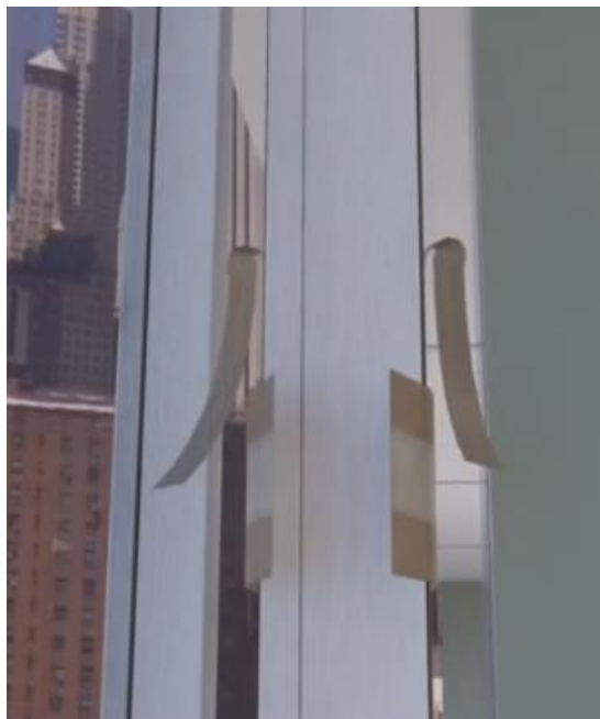
Figure J: Mullion Mate® Pro FR in location removing gasket release sheet and straps
