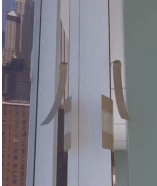
Figure B: Mullion Mate ® in location removing gasket release sheet and strap
