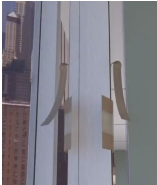
Figure B: Mullion Mate® PLUS in location removing gasket release sheet and strap
