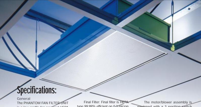
The PHANTOM FAN FILTER UNIT is a low profile fan powered HEPA filter module manufactured by GORDON CLEANROOM PRODUCTS, Shreveport, Louisiana.
