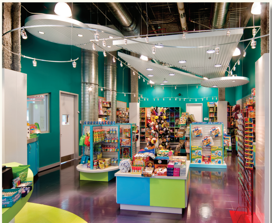
Triangular and Circular Cloud Ceilings with ALPRO Corrugated Panels and Perimeter Trims, Face-Attached to Concealed Suspension System
