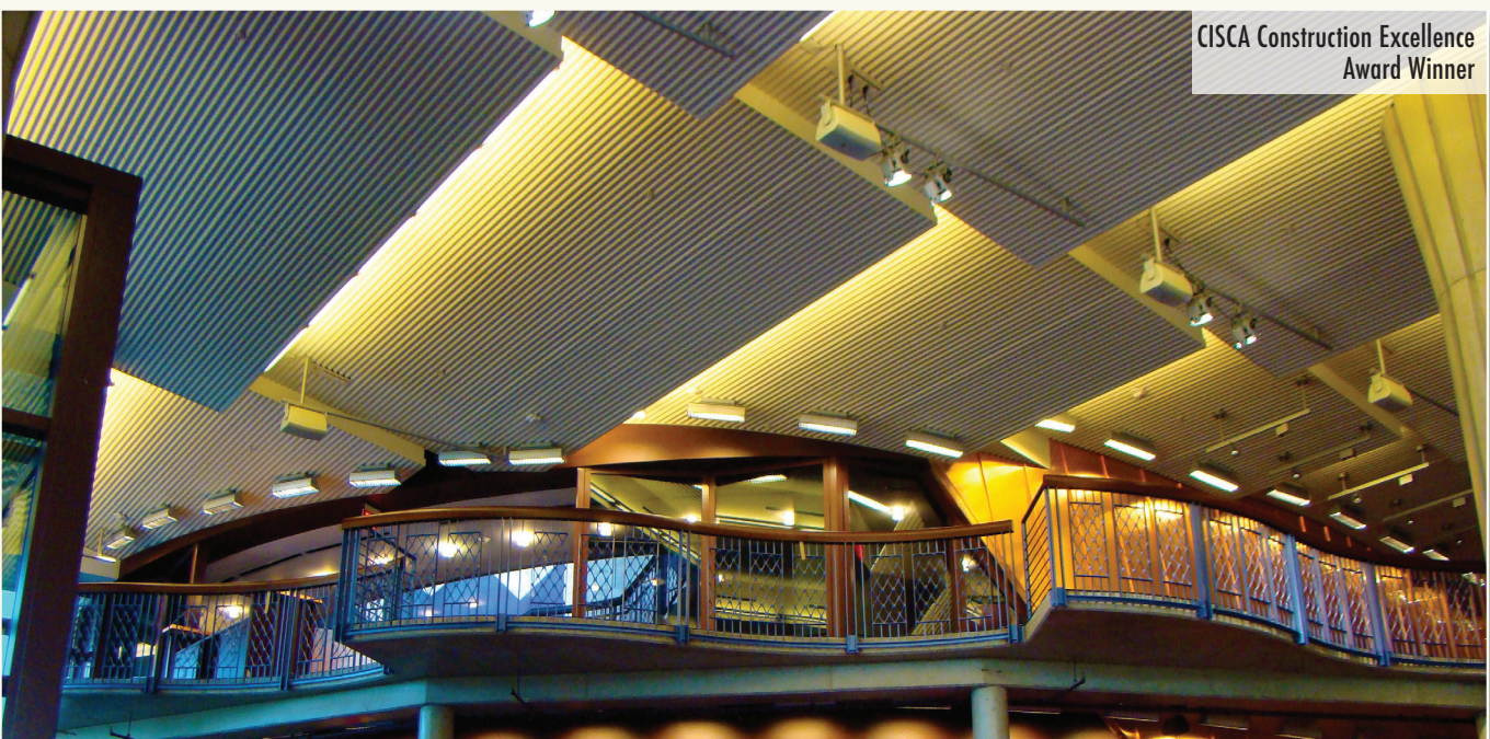
Cloud Ceilings with ALPRO Corrugated Panels and Perimeter Trims, Face-Attached to Concealed Suspension System
