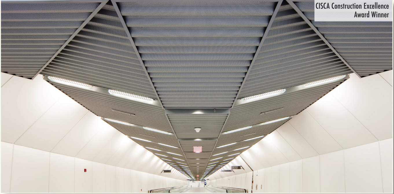
Custom Ceilings with ALPRO Factory Mitered Corrugated Panels Face-Attached to Concealed Suspension. Ceilings include Perimeter Trims, Integrated Lights, and Sprinklers.
