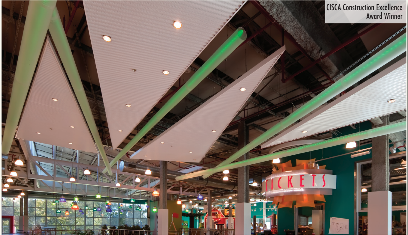
Triangular and Circular Cloud Ceilings with ALPRO Corrugated Panels and Perimeter Trims, Face-Attached to Concealed Suspension System
